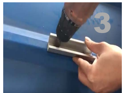
Fasten the mini rail with metal sheet roof with 2pcs st6.3*25 tapping screw.
